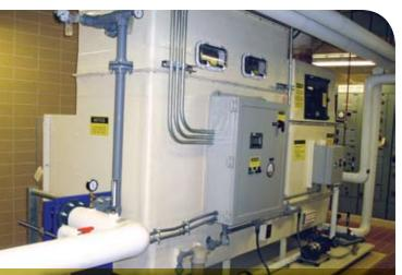
Liquid desiccant units like this Kathabar installation can be used for a wide variety of industrial process and comfort dehumidification applications. Photo courtesy Niagara Blower Company.
