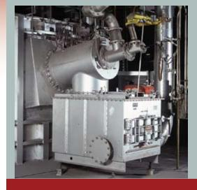
Bloom regenerative burners on an aluminum melting furnace improve efficiency by capturing heat that would otherwise be lost to the burner exhaust. Photo courtesy Bloom Engineering.
