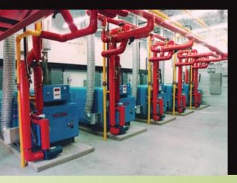
Installation of multiple units allows redundancy for service outages and allows units to be staged on to meet changing electrical demand. Photo courtesy Tecogen.
