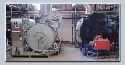
Coil tube boilers fit in well with existing plant units. Here a 450 bhp Vapor Power Circulatic<sup>®</sup> horizontal coil tube boiler stands alongside a 250 bhp firetube boiler. Note also the similar footprint for the larger capacity coil tube boiler. Photo courtesy Vapor Power.
