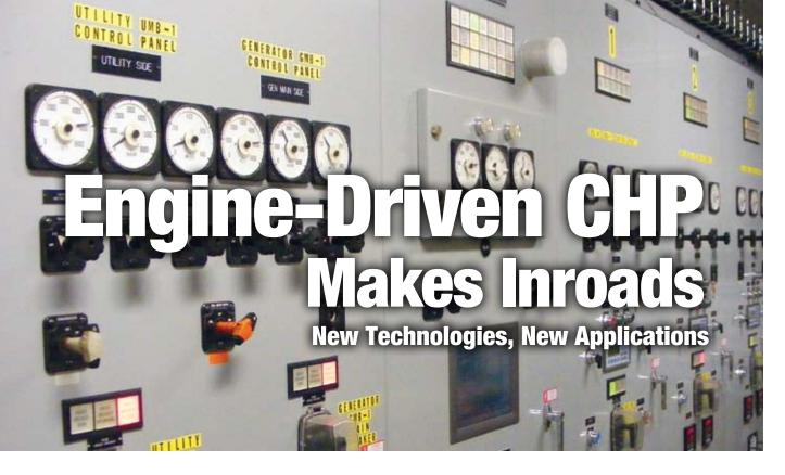
**FOR THE RIGHT INDUSTRIAL** application – and there are many of them – a combined heat and power (CHP) engine system fueled with natural gas is an ideal package. The concept is simple. A rugged internal combustion engine turns an electric generator. Engine byproduct heat generates hot water. In this way, the fuel utilization is far more efficient than electricity and water heating fuel purchased separately.
