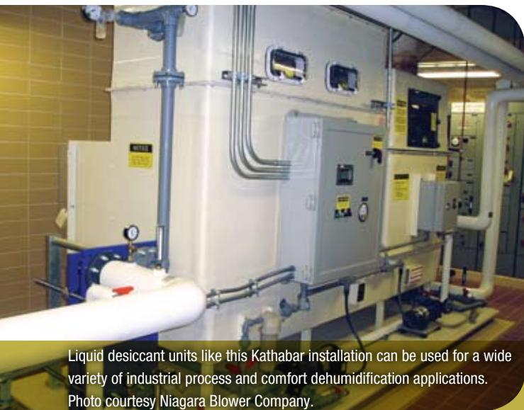
Liquid desiccant units like this Kathabar installation can be used for a wide variety of industrial process and comfort dehumidification applications. Photo courtesy Niagara Blower Company.
